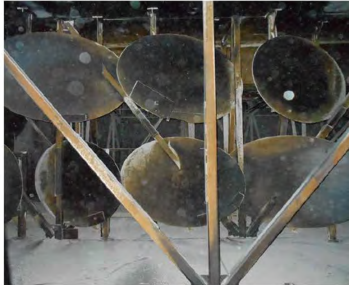
Economizer outlet, compilation photo of mixer plates (flow is into page)
